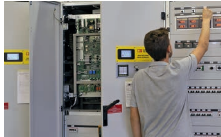
FAT, Start-up & Commissioning
